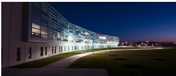
Advanced Technology Research Facility
